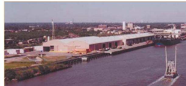
The new Rubb dockside warehousing at Port Arthur, USA
