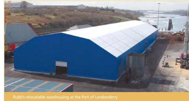
Rubb's relocatable warehousing at the Port of Londonderry
