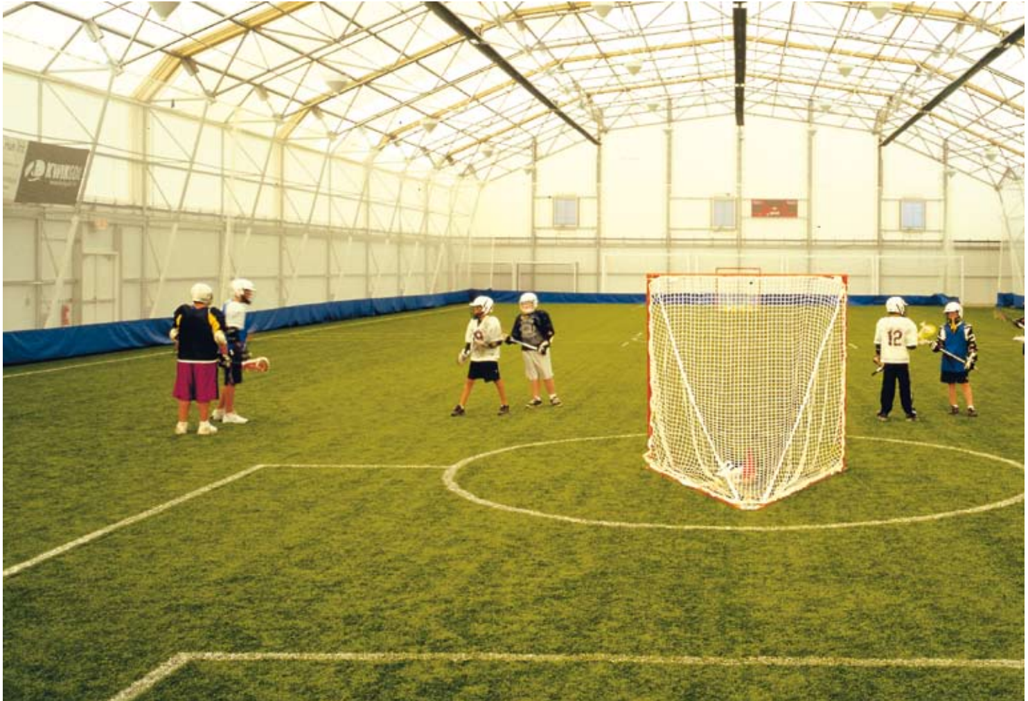
This sports facility, which was originally built in Boston, Massachusetts, was relocated, re-erected and lengthened in York, Maine, USA
